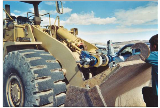
Line Boring A Set Of Digger Bucket Pivot Bearings Approx 60mm Ø
